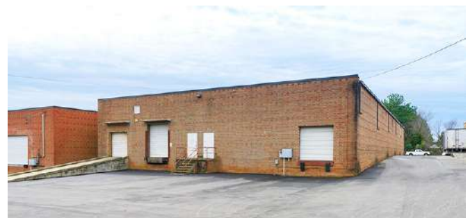
Newly paved truck court
