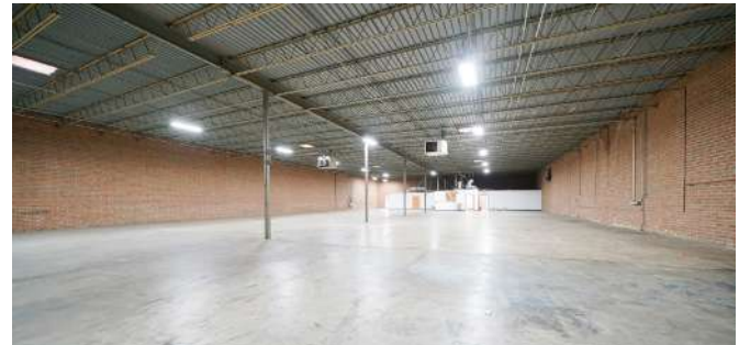
Warehouse: new LED lighting
