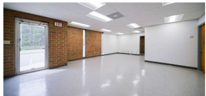
Front Showroom: new flooring, LED lights, paint
