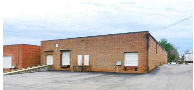
Newly paved truck court
