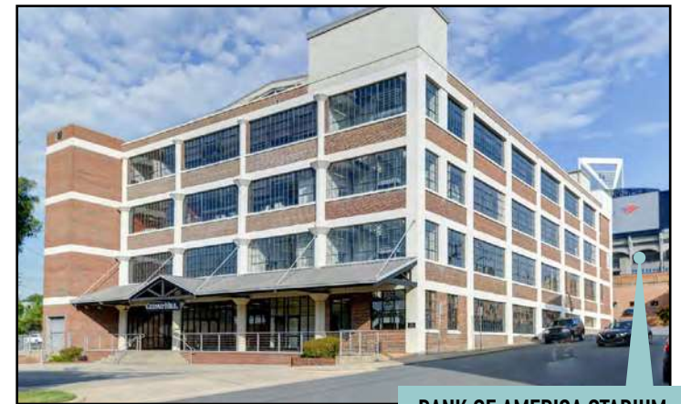
BANK OF AMERICA STADIUM
