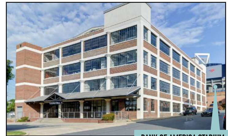
BANK OF AMERICA STADIUM
